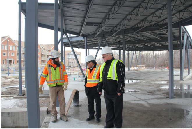
Roman Lim and Deacon Gerry inspect the progress of the Church construction
